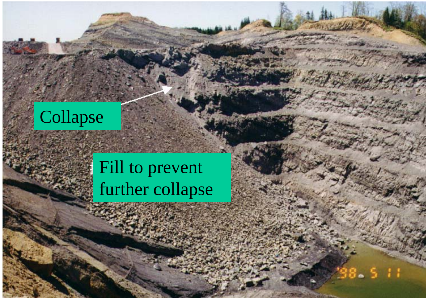
Rock slope collapse at Sunago Coal Mine. A bench is 10 m high, volume is 13,500 m 3
